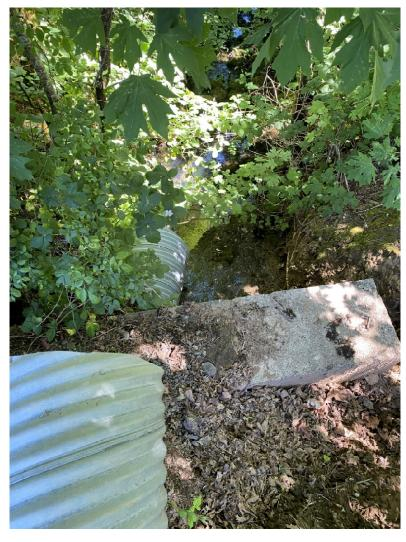
Photo 2: Photo of existing culvert that conveys flow from Spring Brook across Southern Pacific Railroad to the south. Image taken 6/6/2024.
